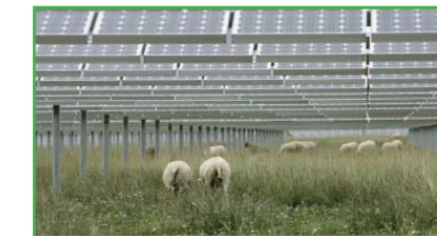
Farm solar generation system
