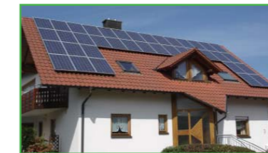
Off-grid home solar system
